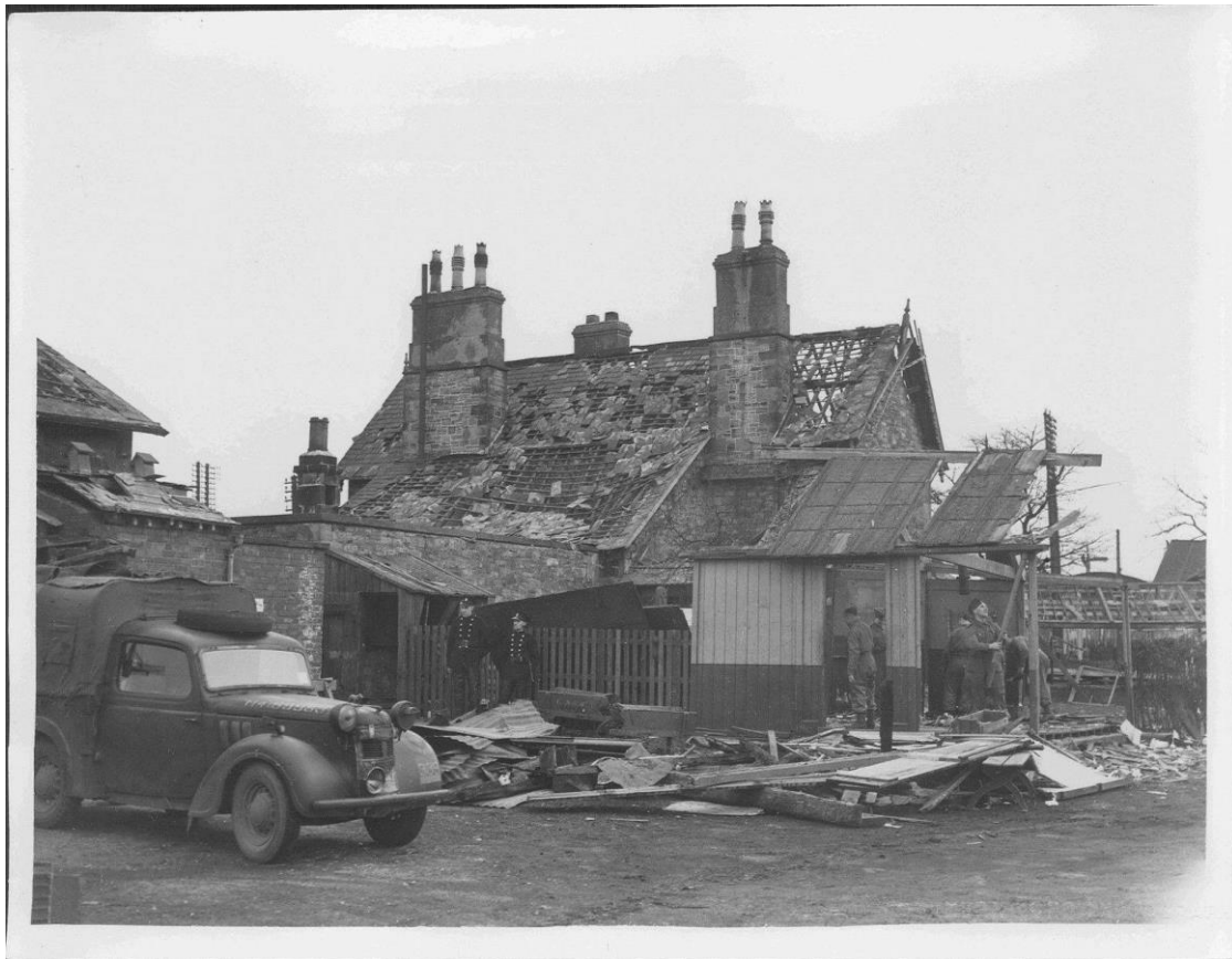
The Station from the rear:
